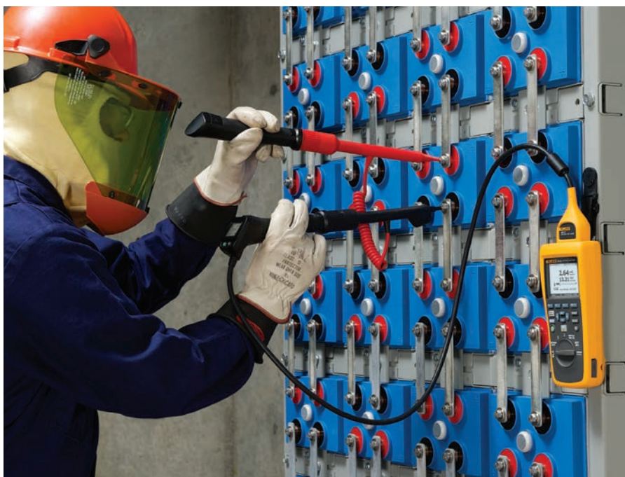
Measuring ohmic values in sequence mode
