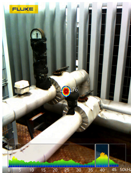
Leak detection on a pipeline
